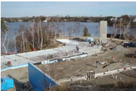
Vale Inco Living with Lakes Centre Construction Progress: Oct, through Nov - in floor radiant pipes are installed, concrete floors are poured, vapour barriers installed and the buildings' shape is now evident.
